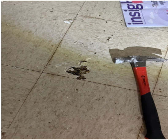
Photo 1 – View of 12"x12" beige floor tile with associated asbestos containing black mastic.
